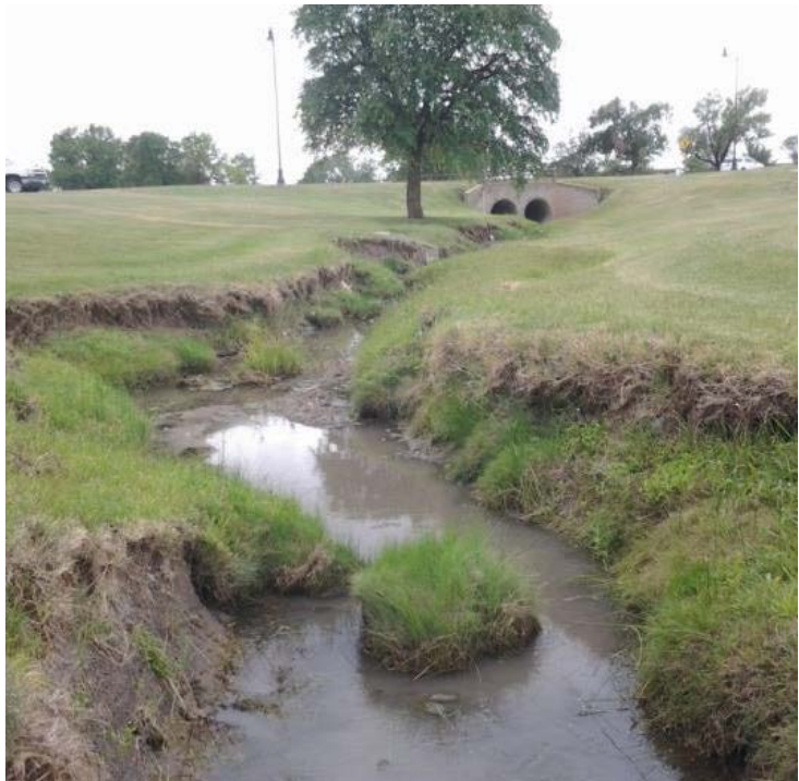
Figure 14: Bank sloughing along a mowed stream.
