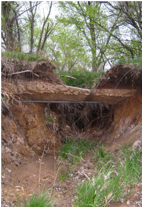
Figure 13: Uncovered Utilities at MAFB
