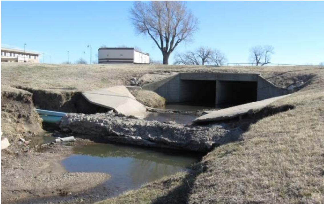
Figure 12: Stream Infrastructure Erosion at MAFB
